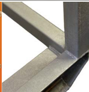
Hot Dip galvanized frame.
