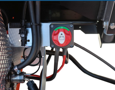
Main battery switch
