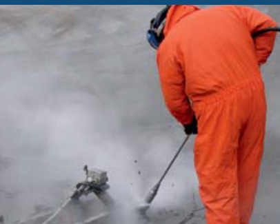
Removing concrete
